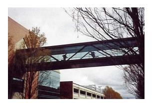
Illustration 1. A sky-bridge is an enclosed horizontal passageway spanning from one building to another building that allows persons to walk from one building to a neighboring building without exiting either building.
